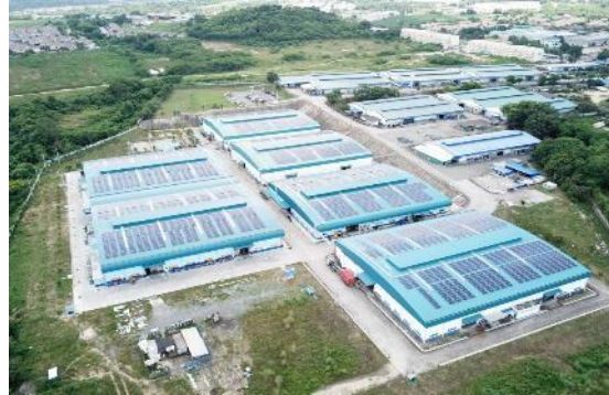
SOLAR ROOFTOP 1 Project Sriracha, Chonburi
