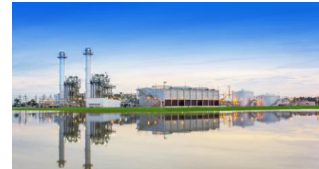
Co-gen 1 project (COD projects)
